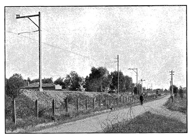
NEW TYPE OF OVERHEAD MAST STRUCTURE MANUFACTURED FROM OLD RAILWAY RAILS. McLeod—Mont Park.
