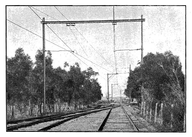
NEW TYPE OF OVERHEAD MAST STRUCTURE MANUFACTURED FROM OLD RAILWAY RAILS. McLeod—Mont Park.
